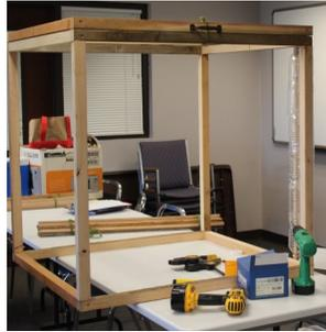
2. Connect two of the "windows" with the uprights. Use 2 1/2" or 3" screws. Place screws off center so they do not interfere with leg installation.
